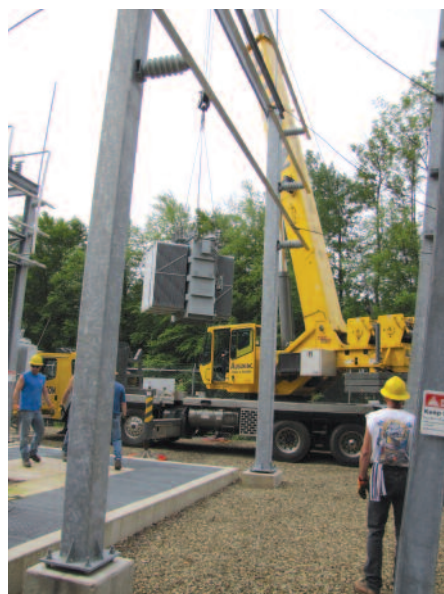
NO EASY TASK: Moving a 27,300-pound transformer requires special equipment.
