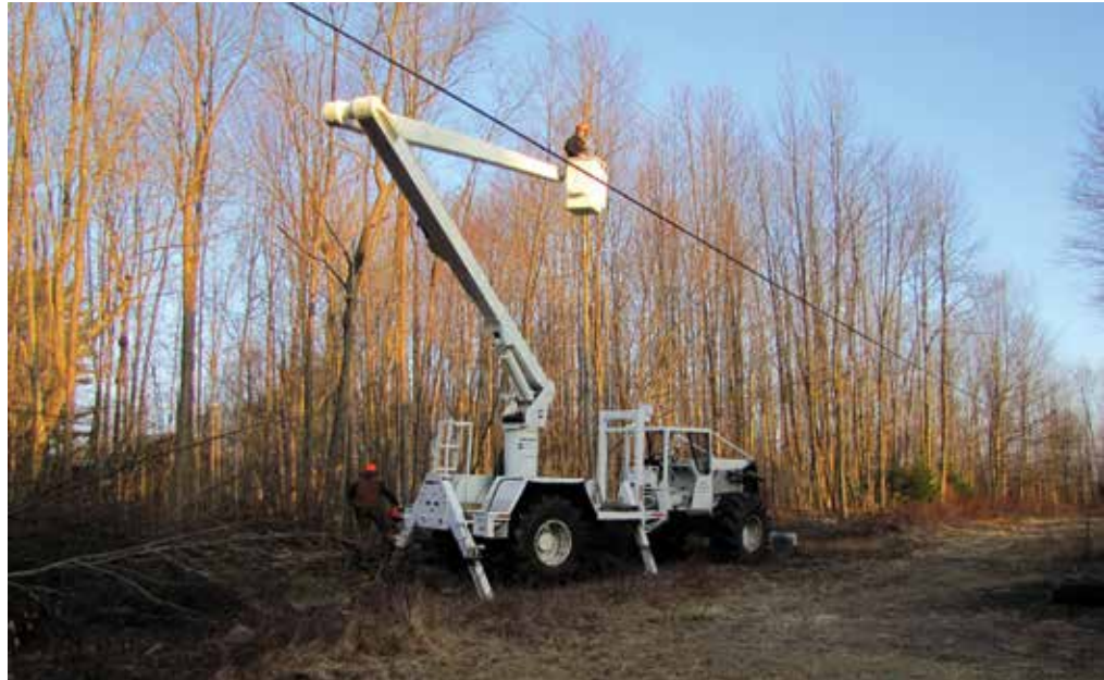
EFFICIENT EQUIPMENT: The skidder bucket purchased by Spako Tree Service is a valuable piece of equipment that makes our right-of-way maintenance much more efficient.
